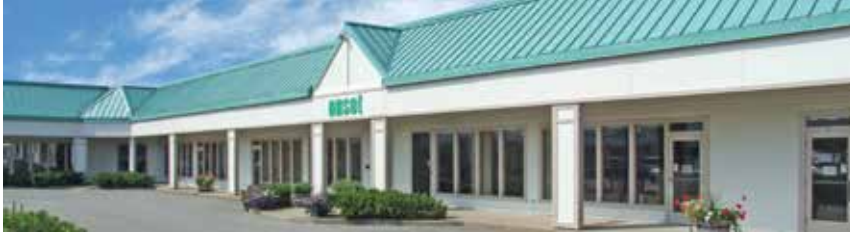
Onset headquarters, Cape Cod, MA
